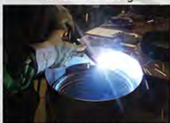
Welding Interior Pipe to Housing
