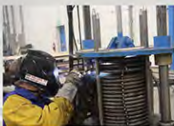
Compressing & Welding Pancake Bracing
