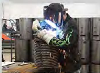
Welding Additional Bracing
