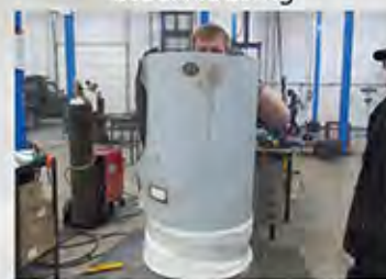
Installing Stainless Steel Housing
